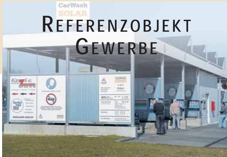
Neubau Car Wash Solar, Frauenfeldstrasse 21, Winterthur
