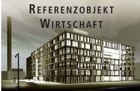
Siemens Building Systems, Zug
